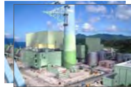
Lungmen 1&2 94% complete Pre-op testing
