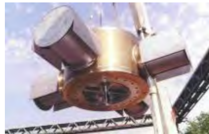
drywell to wetwell vacuum breaker test
